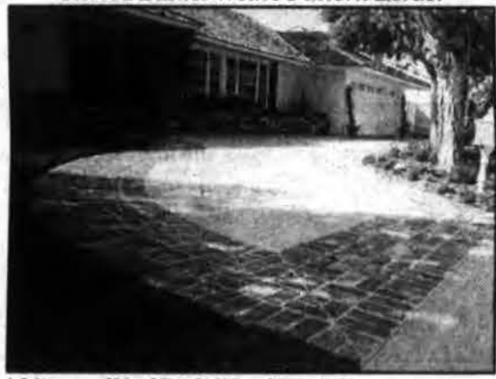
A Mixture of Used Brick &amp; Sand Finish Concrete Driveway
